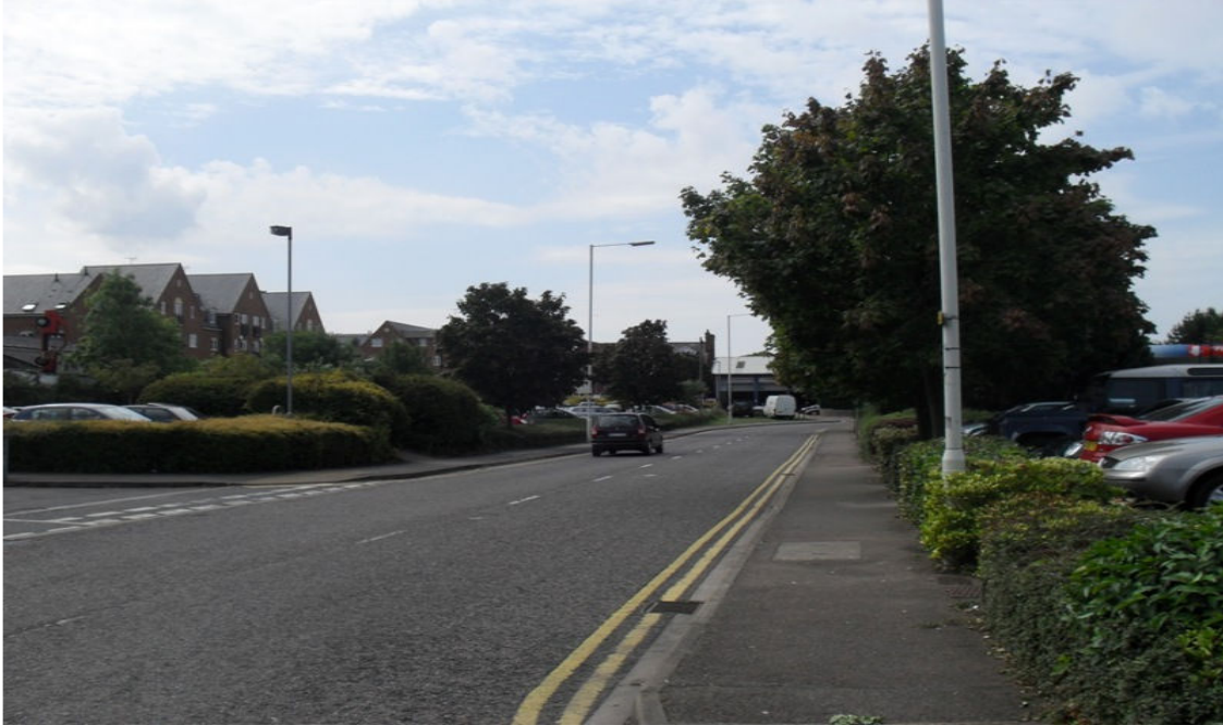
Middle Exit looking south
